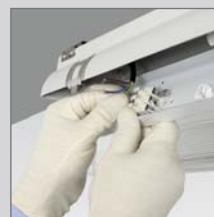
4. disconnect gear tray
