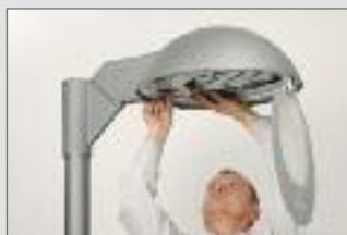
2. Fold the cover down. A further twist-lock catch locks the gear tray
